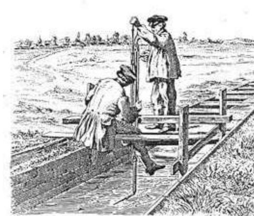
Figure 7. Technicians using a Pitot-Darcy tube (Darcy and Bazin, 1865).
